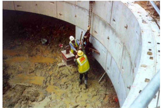
Segmental shaft sinking at Reskadinnick, Camborne, Cornwall
