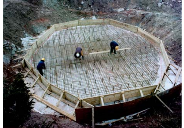
Fixing reinforcement to a shaft cover slab, Nr Redruth, Cornwall
