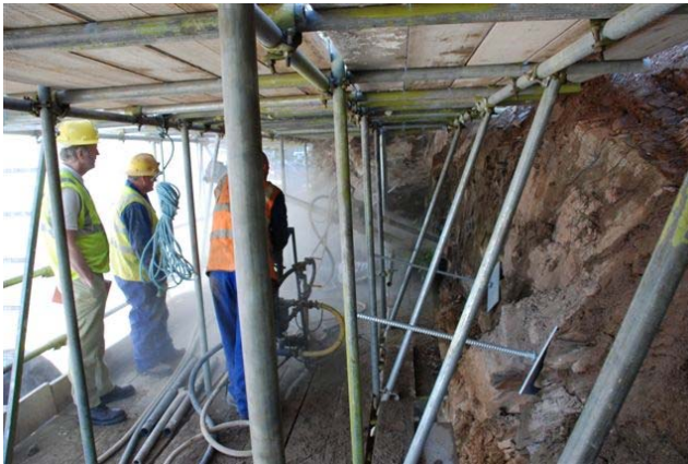
Rock bolting in Looe, Cornwall
