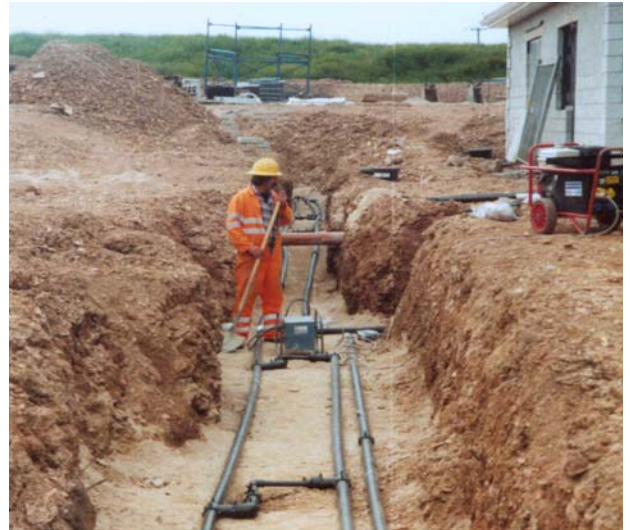
Geothermal heat pump system installation in Tolvaddon, Cornwall
