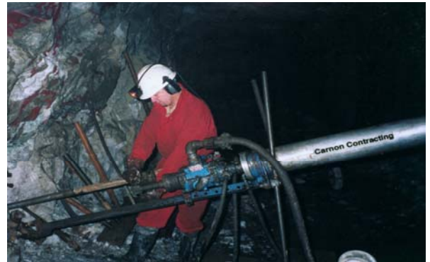
Underground drilling in Greece
