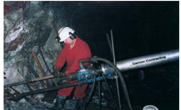
Underground drilling in Greece
