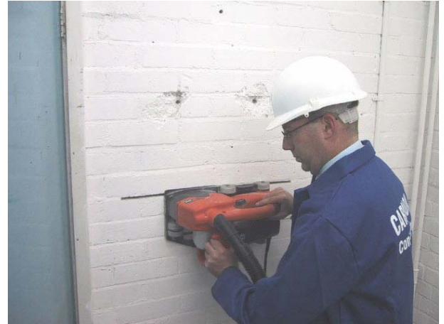
Chasing machine being used for crack repairs
